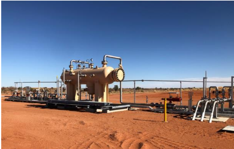
INFRASTRUCTURE IN PLACE
