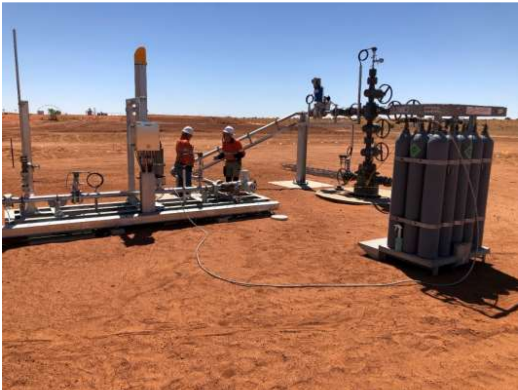
Nitrogen purge operations during commissioning at Vali-1
