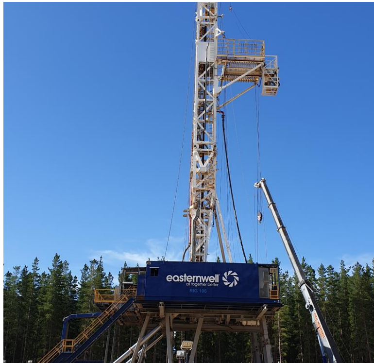
Figure 1: Easternwell 106 on site at Nangwarry-1
